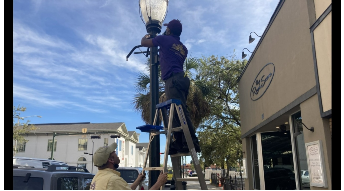
Ambassadors John and Clayvon are hard at work hanging holiday lights. Putting up these lights is a yearly tradition that make the streets look spectacular at night time.
