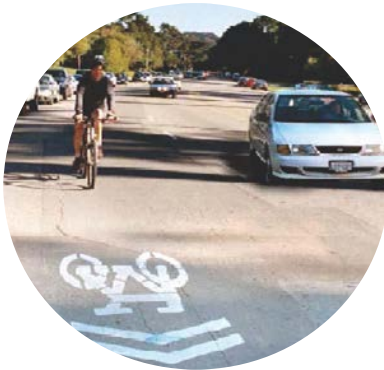
Shared Use Markings
