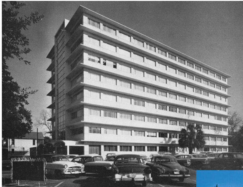
The current rehabilitation project restored the exterior to its original appearance by repairing the bands of windows, restoring the main entry, and refreshing the stucco walls and canopies. The main lobby was restored to showcase the monumental cantilevered stair, terrazzo floors, planter and fountain, and stone veneer walls.
