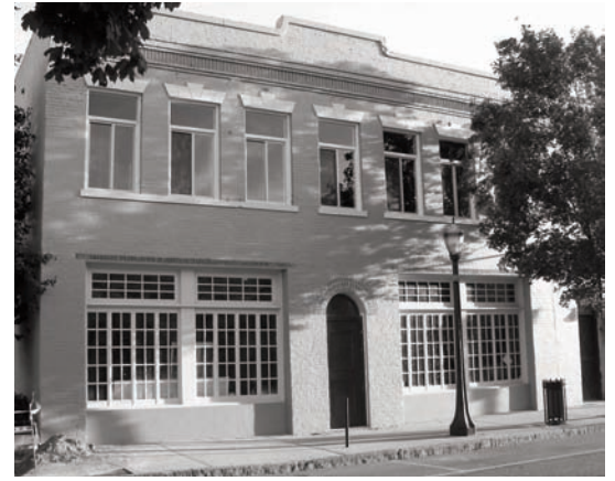
The conversion of the 1860s horse-drawn carriage company at 709 Dauphin Street will create seven residential units known as Carriage Works . Some of the units will be finished in May.
