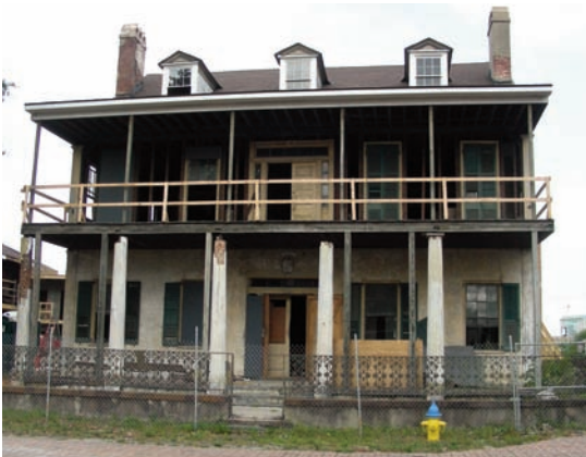
The Hall-Ford House in Fort Conde Village is one of the most beautiful buildings being renovated by developer Larry Posner . The structure is considered one of the most significant historic houses in Mobile and will be converted into a nine-room bed and breakfast with meeting space.
