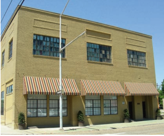
The building at 308 St. Louis Street has been a car dealer, a restaurant supply company and now urban residences. 21 residential units now make up St. Louis Lofts .
