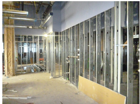
View of unit framing of residential units
