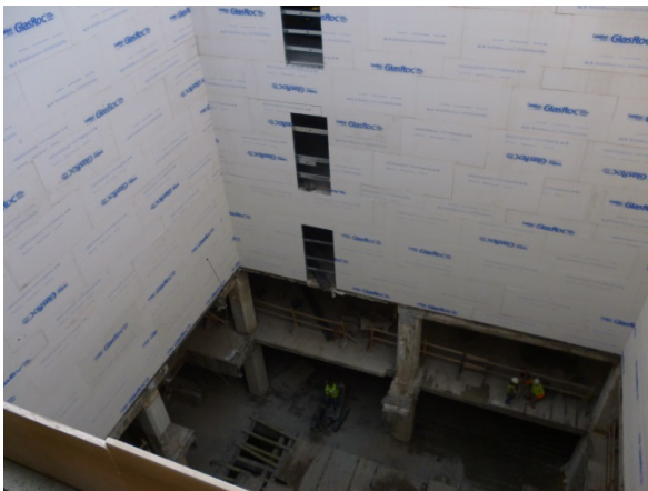
View of interior lightwell added to center of structure by cutting through each floor plate to add required windows to the new residential units
